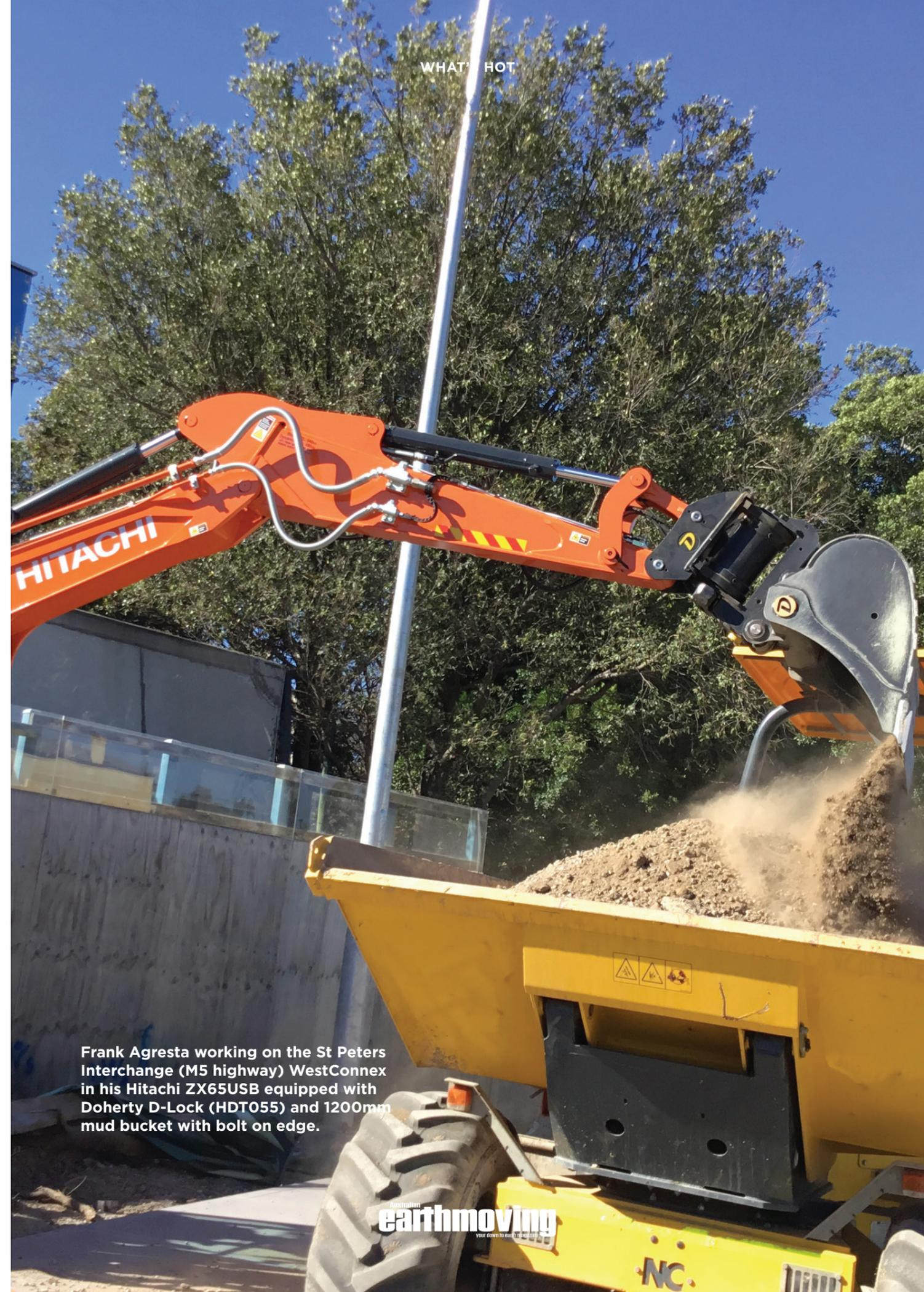
Frank Agresta working on the St Peters Interchange (M5 highway) WestConnex in his Hitachi ZX65USB equipped with Doherty D-Lock (HDT055) and 1200mm mud bucket with bolt on edge.
