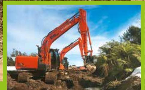
**The excavation of a storm water outfall utilising the Snaplock+ Tilt and Doherty 1.8-wide cleaning bucket along with the Leica 3D system**
